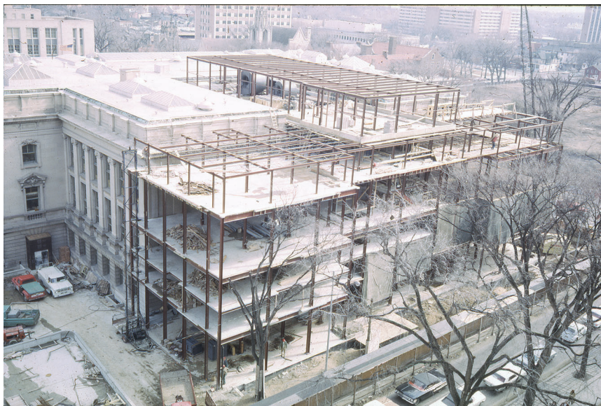
A T-shaped addition to the society headquarters under construction, 1967. (WHi Image ID 98620)
