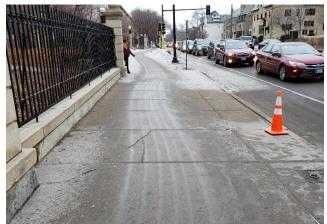
In this photo, notice the lines showing effective anti-icing application on the sidewalk.
