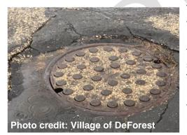
Open pick holes in manhole covers are points where salt-rich stormwater can enter the wastewater sewer.
