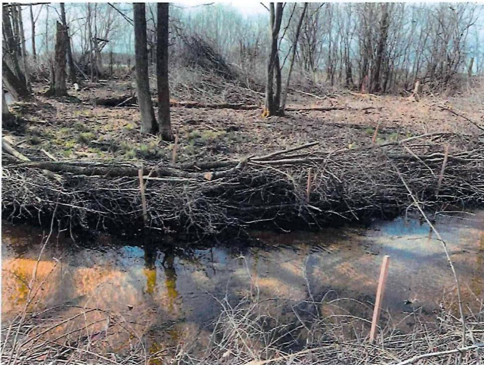
Figure 5. Brush bundles are placed along banks of the river to promote natural narrowing and deepening of the channel. A narrower and deeper channel helps improve floodplain connectivity, wetland conditions, and native brook trout habitat.
