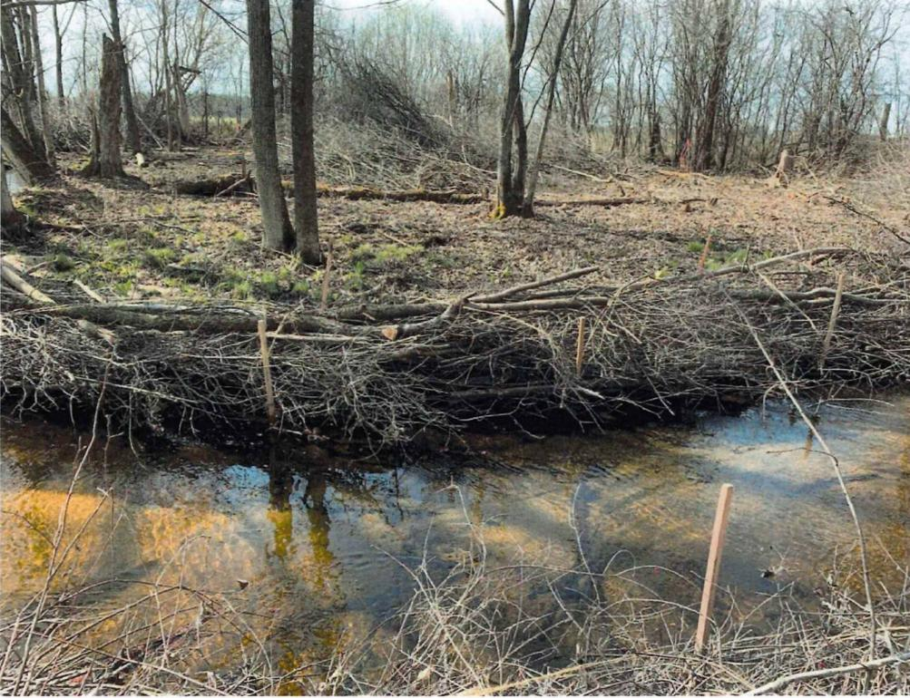
Figure 5. Brush bundles are placed along banks of the river to promote natural narrowing and deepening of the channel. A narrower and deeper channel helps improve floodplain connectivity, wetland conditions, and native brook trout habitat.
