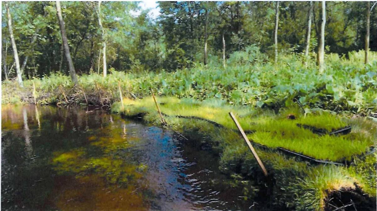
Figure 6. In the first spring after restoration work began, native vegetation is thriving within the floodplain wetlands in areas that have been thinned and where bundles have been placed along the banks of the river channel. Wetland vegetation recolonizing these areas include native ferns, grasses, sedges, rushes, and skunk cabbage.
