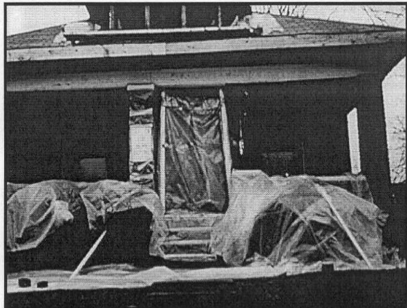
Figure 8.3b Prepare the Worksite With Plastic Sheeting (exterior).
