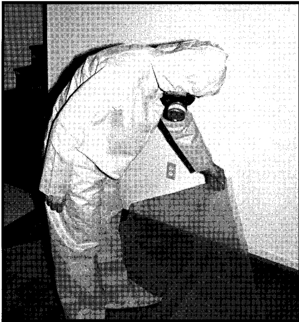
Figure 14.8a Pick Up Corners of Plastic Sheeting.
