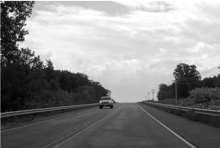
Figure 15: This rural highway bridge has a generous shoulder with a good surface, making it quite suitable for use by experienced adult cyclists.
