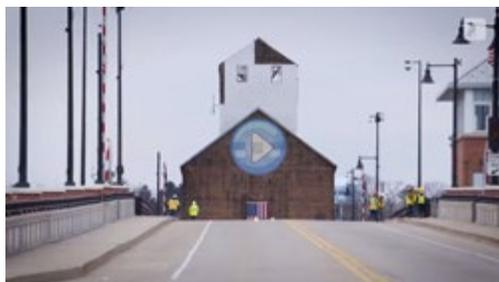
The vehicle used to move the giant structure was a Buckingham BU-173 remote control power unit. This unit is used either manually or by remote control and handles all functions for the load, including raising, lowering, steering, breaking and driving. For this move, the operator carried the wireless remote while walking around the building to observe its progress. Pre-move route preparation included removing traffic lights from the east side of the bridge for clearance.
