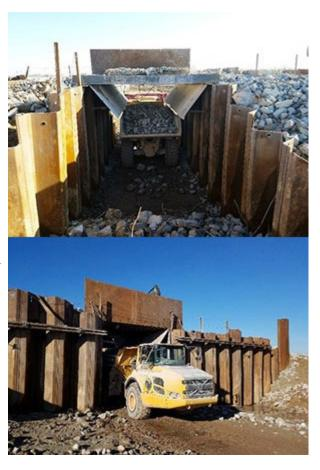
Those sections were then placed on top of grate and operators used vibratory hammer and crusher excavators to separate the concrete from the reinforced steel. The crushed concrete fell through the grate and into the truck staged below before being hauled to an on-site location. The concrete will be used as large, angular breaker run on the WIS 441 Project. Steel is being stockpiled for recycling purposes.
