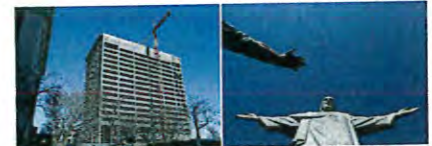
Company taking apart old building
