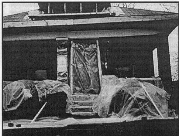
Figure 8.3b Prepare the Worksite With Plastic Sheeting (exterior).
